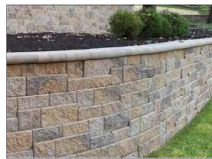
RETAINING WALL RETAINING WALL TO BE SPLIT FACED OR KEYSTONE TYPE. COLOR TO MATCH ABOVE PHOTO
