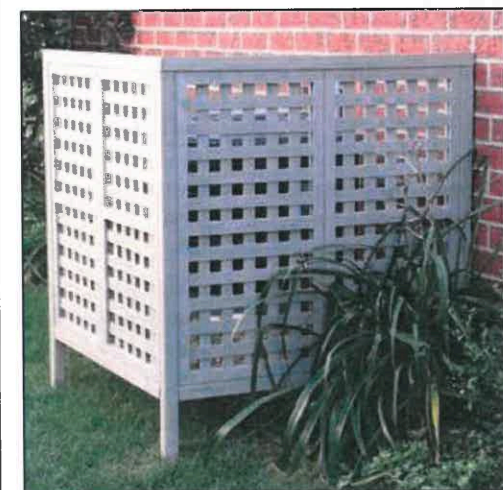
AC UNIT SCREEN: Wood lattice frame components painted to match building wall.
