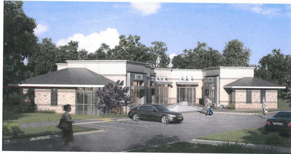
MEDICAL OFFICE BUILDING FACADE, RENDERED
